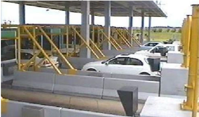
Typical Exit Toll Plaza application:
